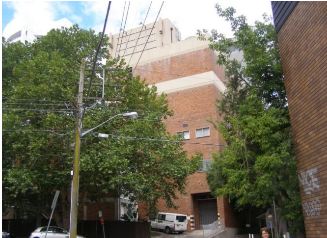
Figure 20 – View of the Telstra exchange building
