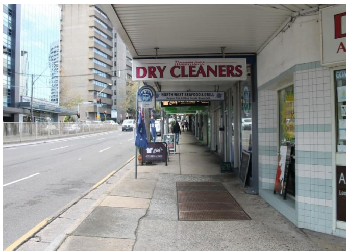
Figure 16 – Existing buildings on the Pacific Highway
